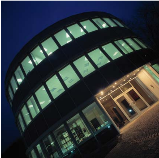
Photo: VARTA Microbattery's Innovation Tower
